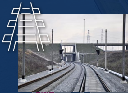
Liefkenshoek Railway Tunnel, Antwerp, Belgium, €690M
