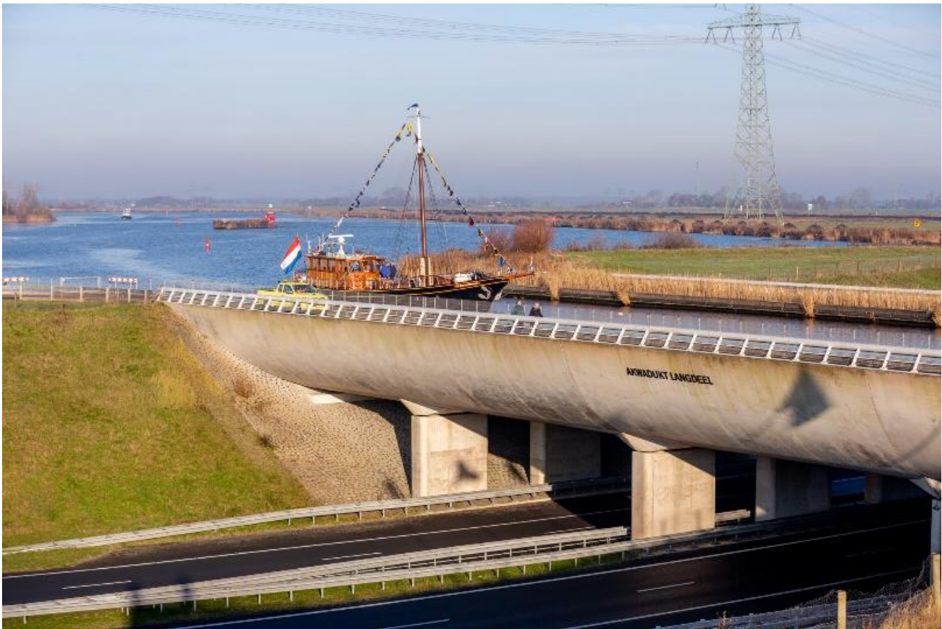
The new aqueduct Langdeel over the N31
