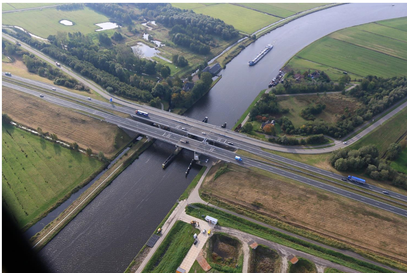
The new Fonejacht bridge with the N31 and a local road passing over the Prinses Margrietkanaal in Friesland
